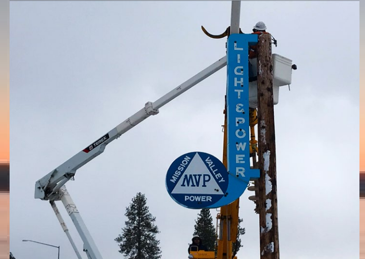
Installing MVP Retro Sign Photo by Shawn Dumont
