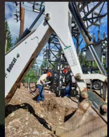
Kerr Substation Work Photo by Jay Fyant
