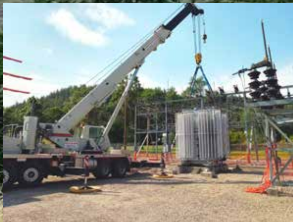
Work at Kerr Substation Photo by Jay Fyant
