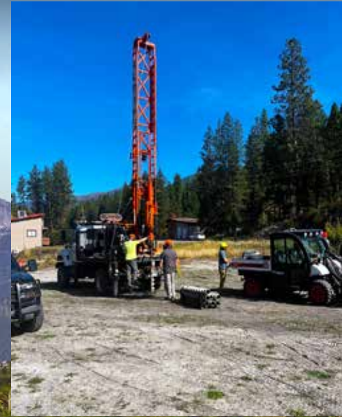
Geo- Testing at Finley Point Sub- station Photo by Bradley Kucera
