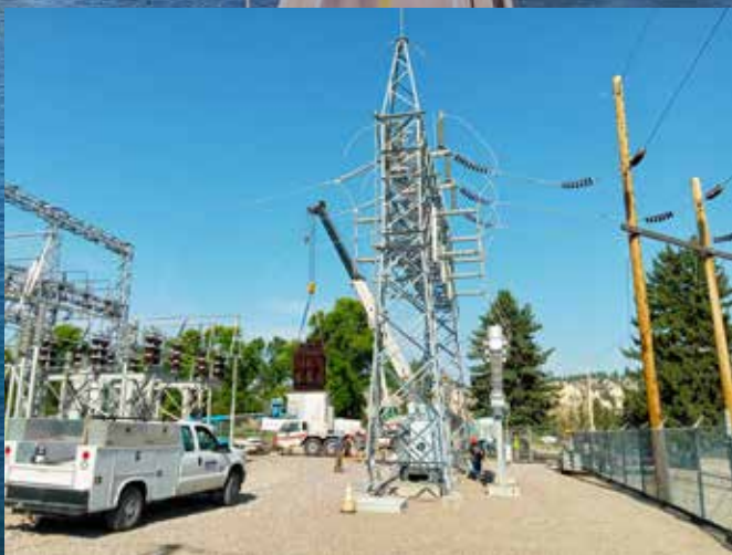
Kerr Substation Work Photo by Jay Fyant
