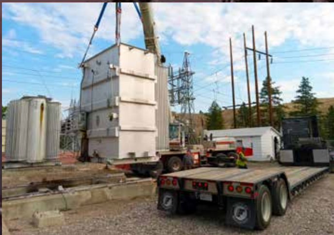
Kerr Substation Work Photo by Jay Fyant
