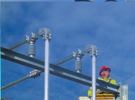
West Shore Substation Work Photo by Jay Fyant
