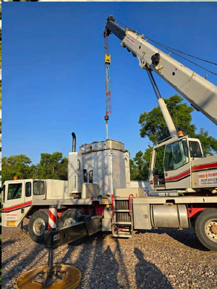
Kerr Substation Work Photo by Jay Fyant
