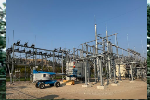
Kerr Substation Work Photo by Zach Felsman
