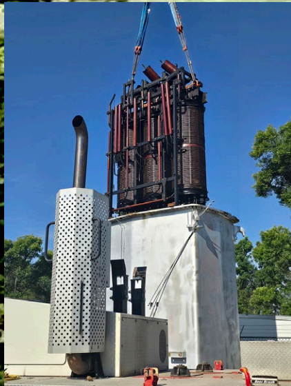
Kerr Substation Work Photo by Jay Fyant
